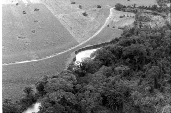
Completely deforested river bank and large bank failure
